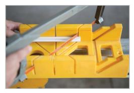
Mitre the two lengths of F-Rail at a 45 degree angle so they meet in the corner.
